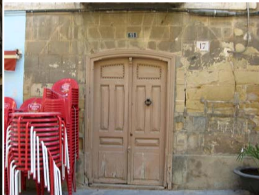
Fachada a C/. Mayor
